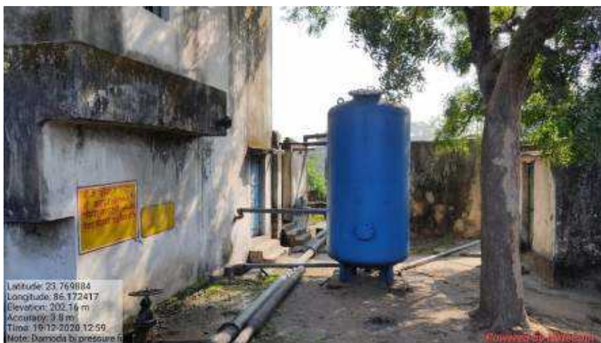
FILTER PLANT IN THE MINE AREA
